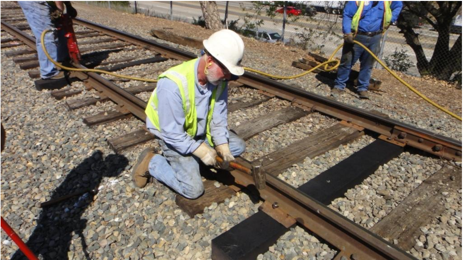
Mike M. drives in by hand one particularly finicky spike
