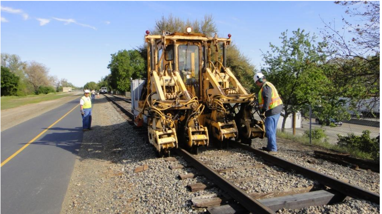
Chris guides from the ground as Steve in the tamper tamps up the new ties.
