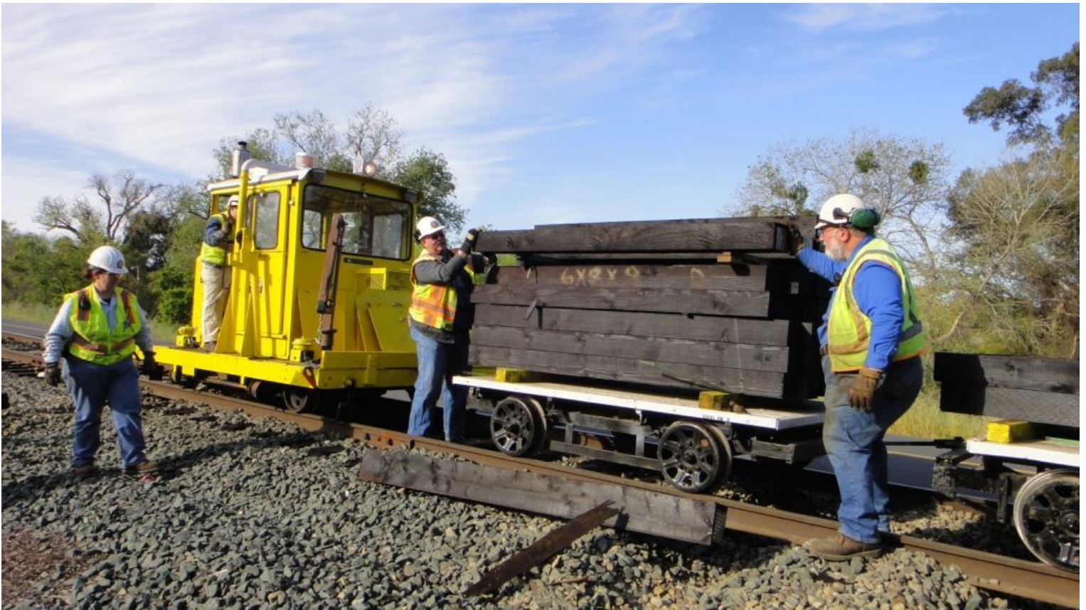
Mike H. pilots the Kalamazoo as Chris and Frank drop ties by the empty cribs.
