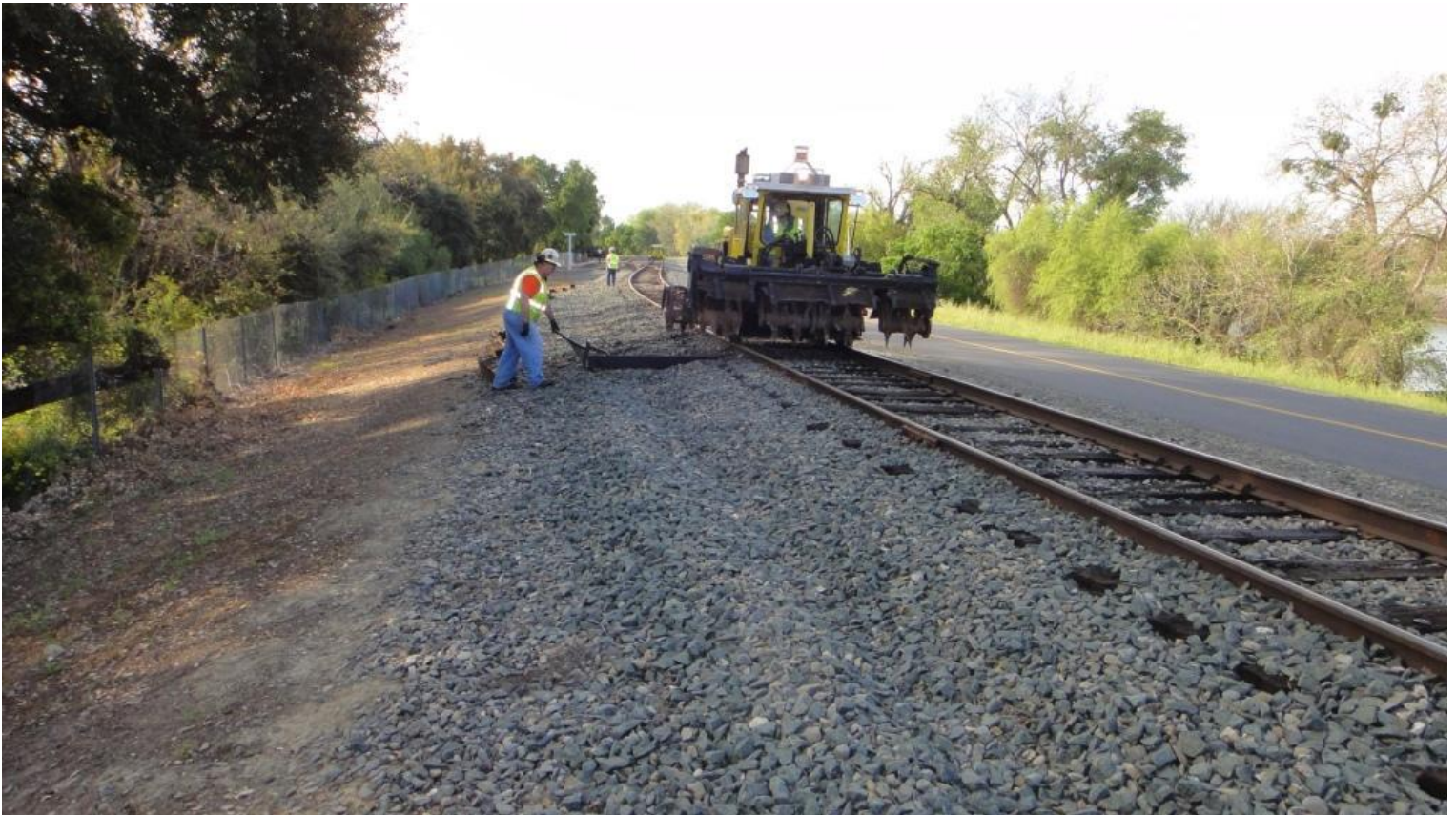
Alan in the scarifier-inserter pulls in a tie as guided by Mike F.
