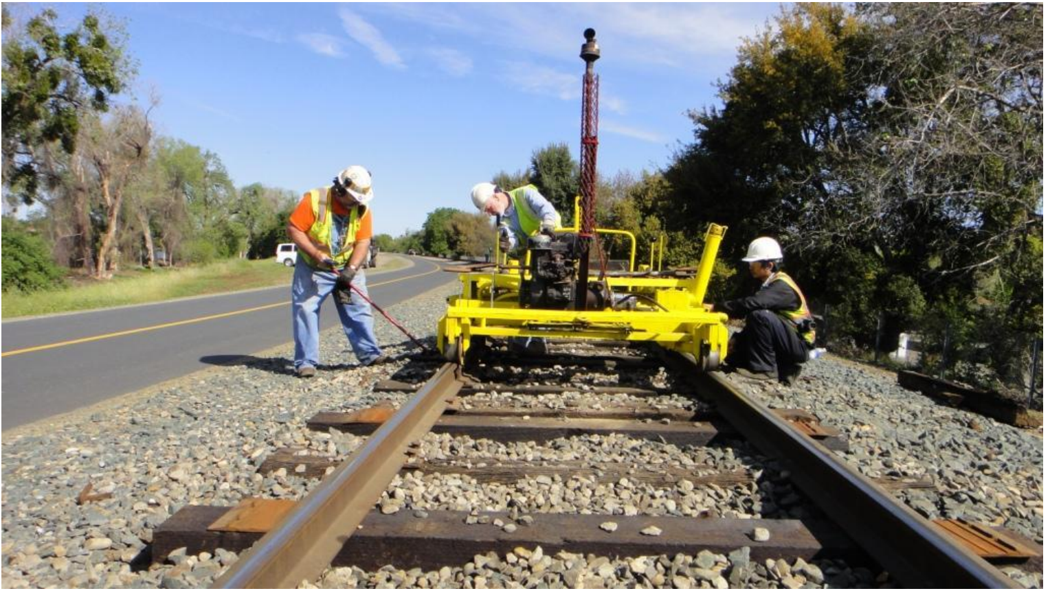
Mike M., at the controls of the rail-lifter, lifts the rail ever so slightly so that Mike F. and Josh can place tie-plates.
