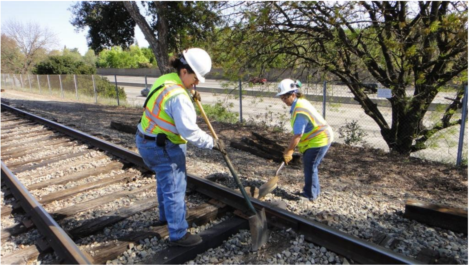
Heather and Pam fill in rock around the newly inserted ties.
