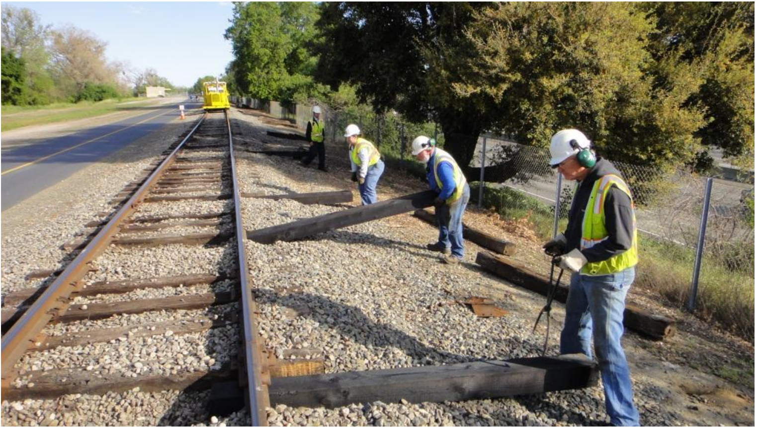
Steve, Frank, Heather, and Josh, our human tie-cranes, position ties for insertion.
